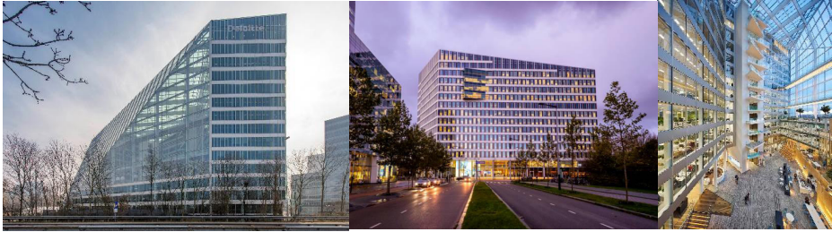
Figure 4. The Edge, Amsterdam. Image courtesy by edge.tech
