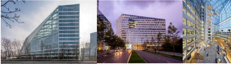
Figure 4. The Edge, Amsterdam. Image courtesy by edge.tech
